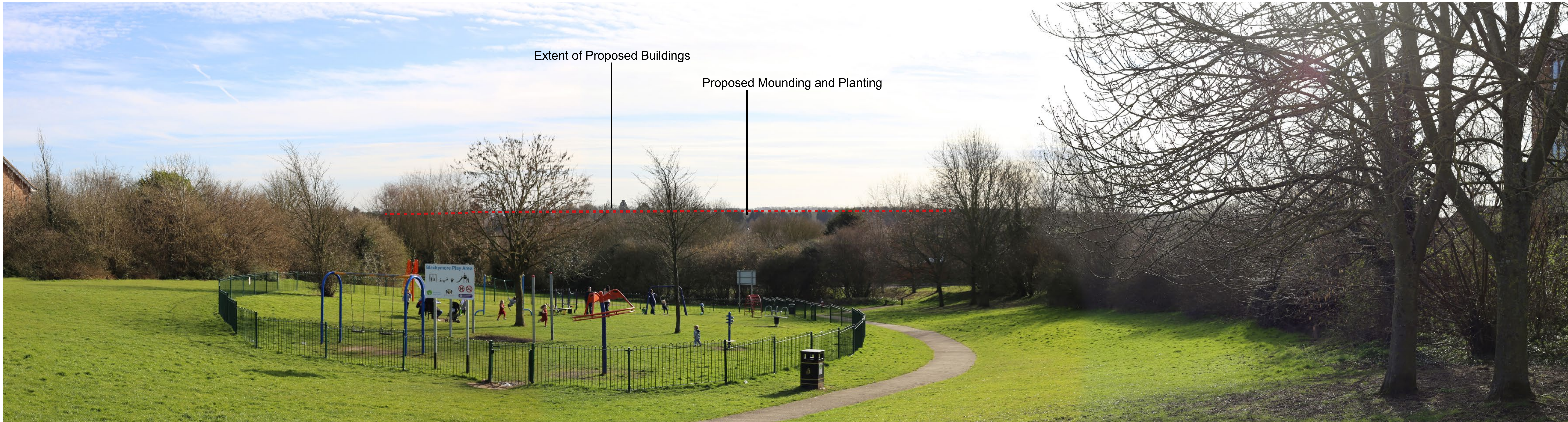
PHOTO VIEWPOINT 22: View upon completion
